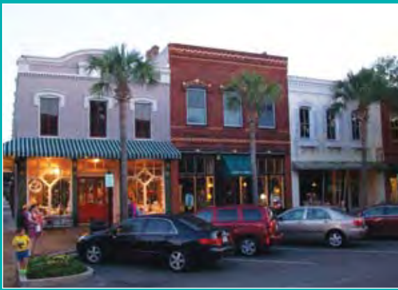
Fernandina Beach, Florida's zoning code allows for residential use on the second floor.
