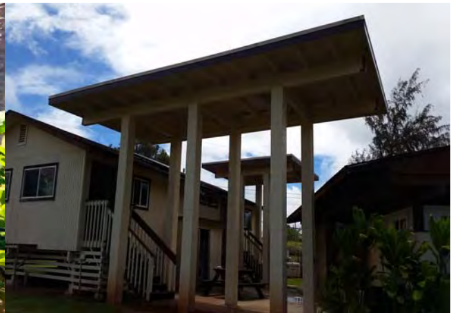
Ho'olehua Fire Station Walkway
